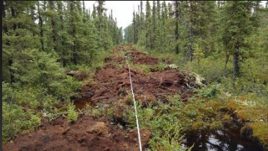
Figure 1. A mounded and planted seismic line in a bog in the Kirby site area
